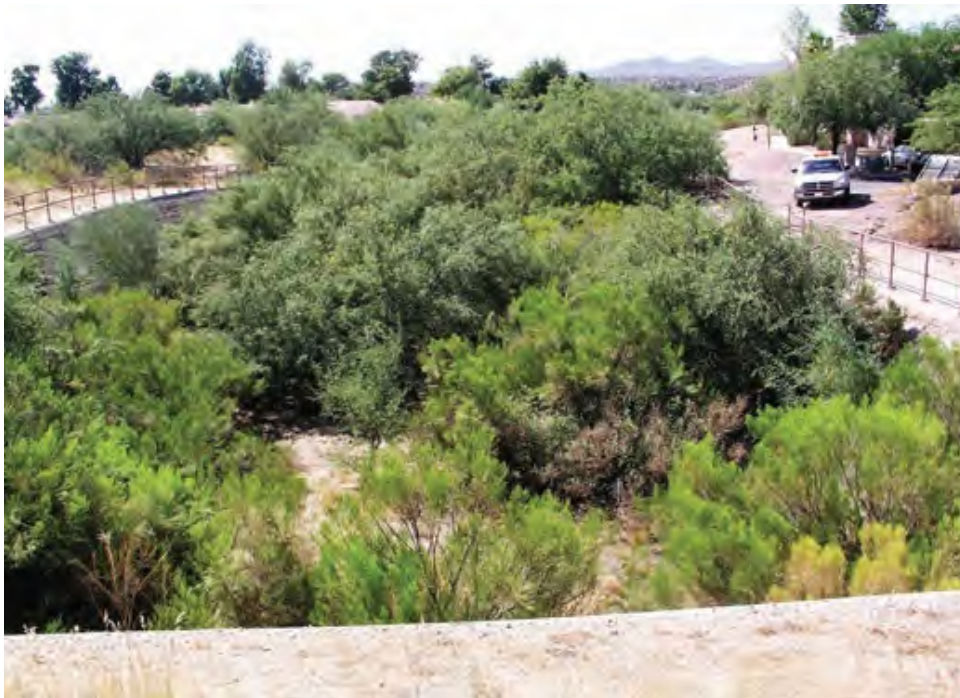
Figure 13. Picture of a constructed channel in Arizona that is overgrown with vegetation (from U.S. Geological Survey Scientific Investigations Report 2006-5108)
